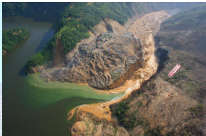
Discharging the Tang-jia-shan quake-lake on June 10, 2008, after the Wenchuan Earthquake in Sichuan, China
